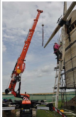
Millwrights remove our windmill's sails as more decay is spotted. Story overleaf
